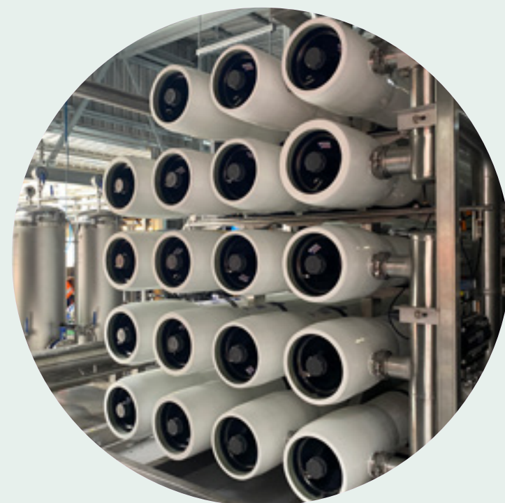
Tooheys recycling plant under construction
